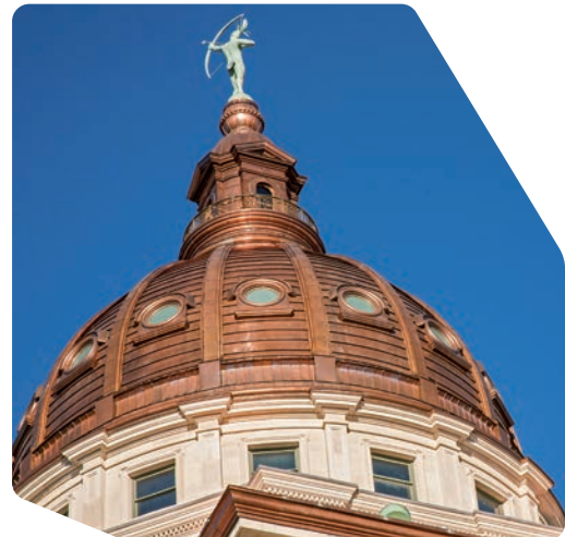
Restoration of Kansas Statehouse (USA)
